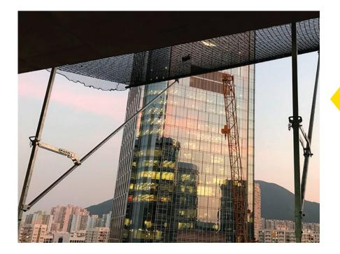
SGB can provide the fall arrest net erected around a building perimeter, to catch both escape of persons and material. SGB Net not only protects site staff working on a building but also the public below from any potential falling debris.
