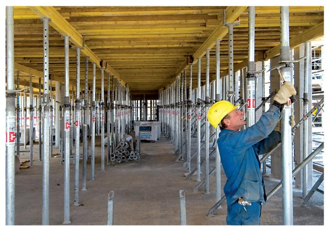
> Stripping is made easier by lowering the forming plane by about 6 cm using the adjustment nut of the steel props
