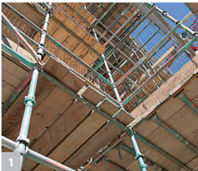
1 Up to 74 kN leg load meaning larger grids and less material
