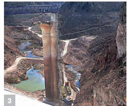
3 High-strength CUPLOK® system allows construction of towers with a height up to 53 m
