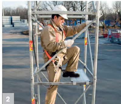
Time-saving and easy handling due to the one-man-assembly utilizing integrated quick-action connector
