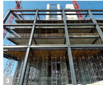
High load capacity of 200 kN per tower even with small base dimensions (1.0 m x 1.0 m)
