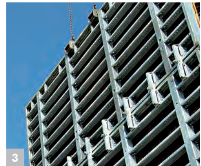
3 Rational forming of larger surface areas without infills and fewer tying points using MANTO XXL panels
