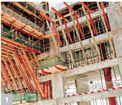
1 Wide range of beam lengths and connectors for all types of heavy shoring and formwork support
