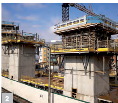
2 Assembles into self-contained, climbing formwork gantries
