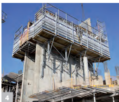
4 Can be used as guided climbing or jump-form system
