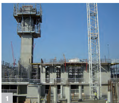
1 Highly adaptable system that supports large panels with safe access platforms
