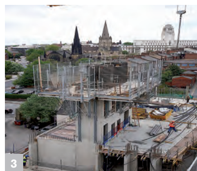
3 Accommodates platform sizes up to 7.2 m long and 2 m wide
