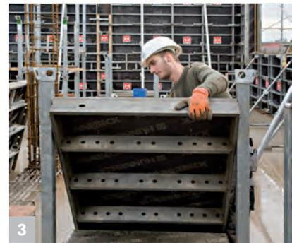
3 Crane-less forming possible due to low weight of basic RASTO and TAKKO panels
