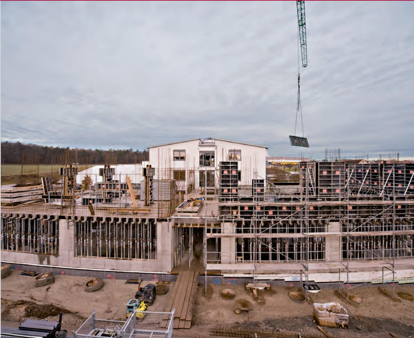
**RASTO-TAKKO is a versatile and crane-independent panel formwork, which offers an ideal solution for small and mid-size projects, especially in residential construction.**
