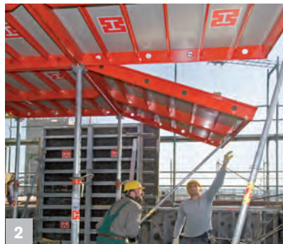
2 Safe forming and stripping up to a height of 3.5 m from the ground in 3 easy working steps
