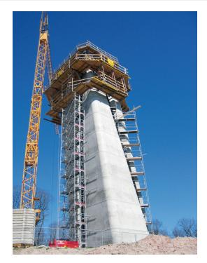
Formwork can be rolled back from concrete by means of move-off unit
