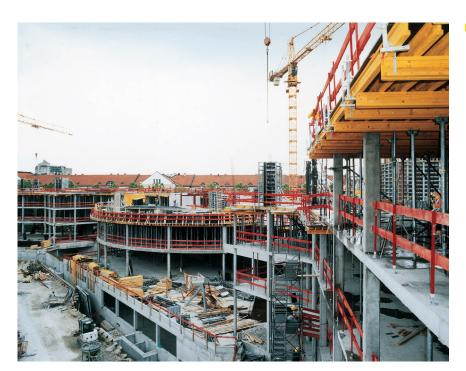
Compatibility with the PROTECTO edge protection system offers extra safety with guardrailing (multiple clamps, posts, etc.)
