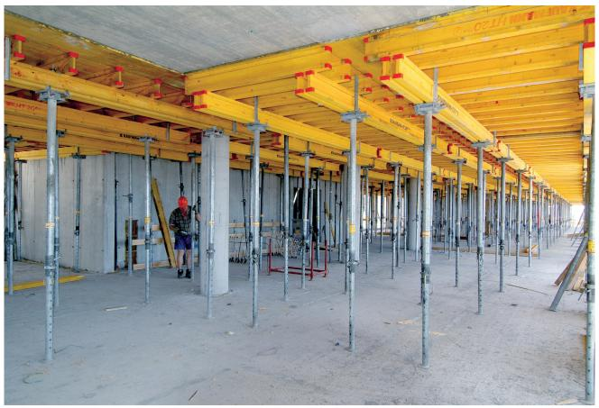
Together with the 21 mm thick plywood form lining, H 20 floor tables can form slabs up to a thickness of 45 cm
