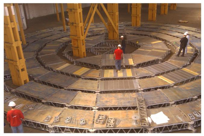
A special solution: Facade walers are used to ensured back anchoring of the horizontal loads and to enable the exact alignment of
