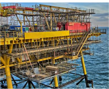
Using QuikDeck®, we can build a temporary work floor for storage and loading of equipment, leaving the often small and heavily contended deck space free – adding flexibility and space during shutdowns, capital projects or decommissioning work.
