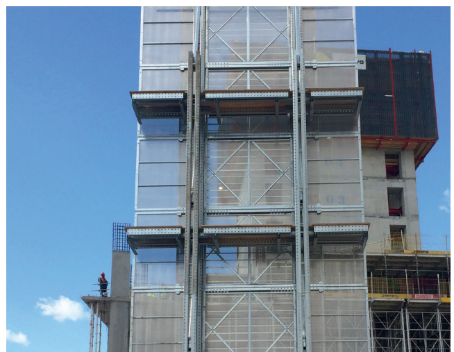
► Multiple floor protection with optional vertical extension
